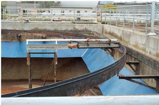
Density Current Baffles
