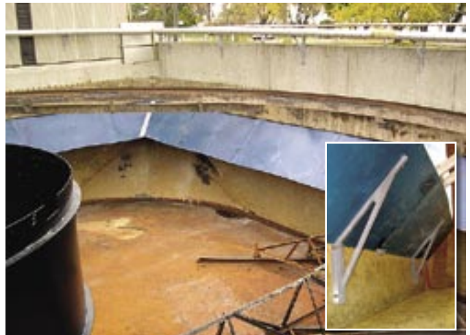
Density Current Baffles
