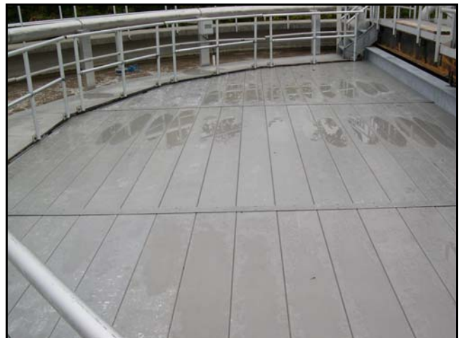
Secondary clarifier cover installation
